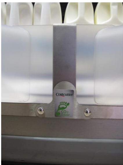
Retro-fit refrigeration scoops reduce consumption by ^10%
