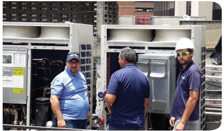
Picture 3. Configuring the VRF systems
